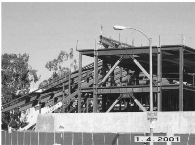
Figure 8.36d. Unbonded brace frame elevation.
