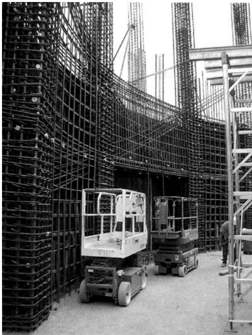
Figure 4.52a. Construction photograph of a diagonally reinforced coupling beam. (Photo courtesy of Mr. Walter Steimle, John A. Martin and Assoc., Los Angeles, CA.)
