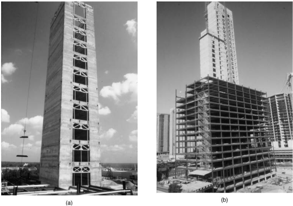
Figure 5.9. Core-supported composite building: (a) concrete core; (b) concrete core encompassed with steel frame.
