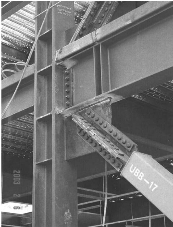
Figure 8.36e. Unbonded brace frame connection (photographs courtesy of Edwin Shlemon, S.E., Associate Partner, ARUP Partners, Los Angeles; CA).
