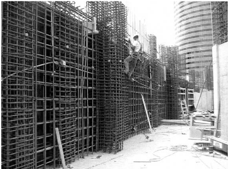
Figure 4.45a. Photograph of a shear wall in seismic zone 4 showing wall-pier and boundary-element reinforcement. (Photo courtesy of Mr. Walter Steimle, John A. Martin and Assoc., Los Angeles, CA.)
