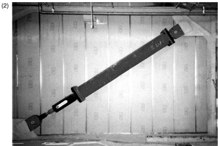
Figure 8.35a. Fluid viscous dampers attached to diagonals: (1) Diagonals with dampers; (2) Close-up of a diagonal; (3) Close-up of a damper. (Photos courtesy of Bob Schneider, Taylor Devices, Inc., New York.)
